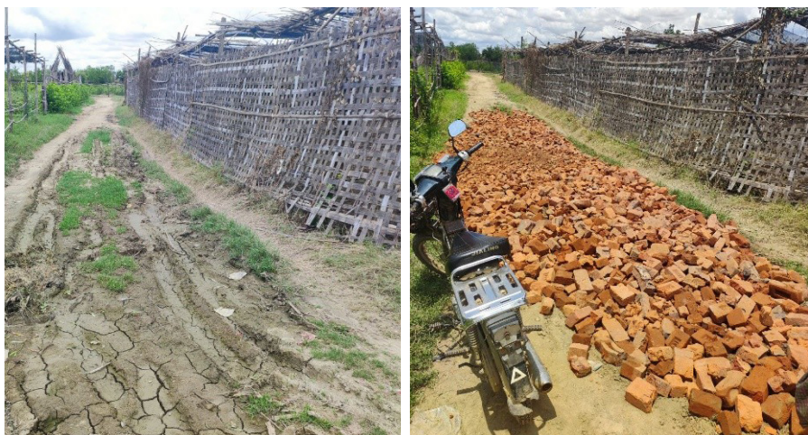
Fig. 17 and Fig. 18 Before (left) and during (right) photos of repair work to the main exit road from a village using funds raised through revolving fund interest, making it easier for residents to flee raids and artillery strikes. Activities such as this enabled the humanitarian committee to build public trust. (photos by Htanaung Collective)
