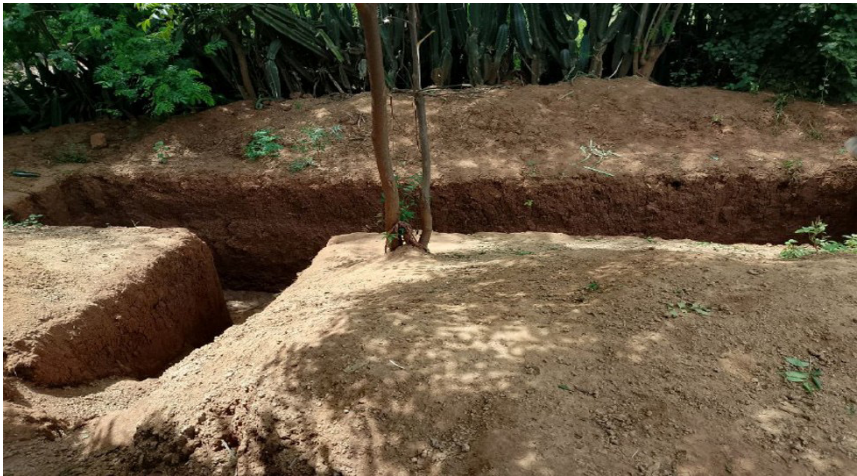
Fig. 9 School bomb shelter under construction (photo by research team)
